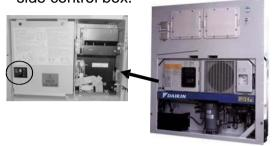
3. Close control box cover and secure latch.
